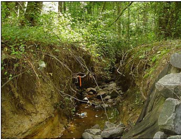
A Reston watershed restoration project intended to repair 14 miles of eroded streams will begin on four miles of Snakeden Branch, left, next month. Reston officials want its streams to look like the stream below, which Wetland Studies and Solutions restored in 2003. (Courtesy Of Reston Association)
